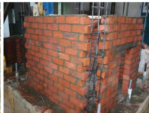
(b) construction of level 1 masonry walls
