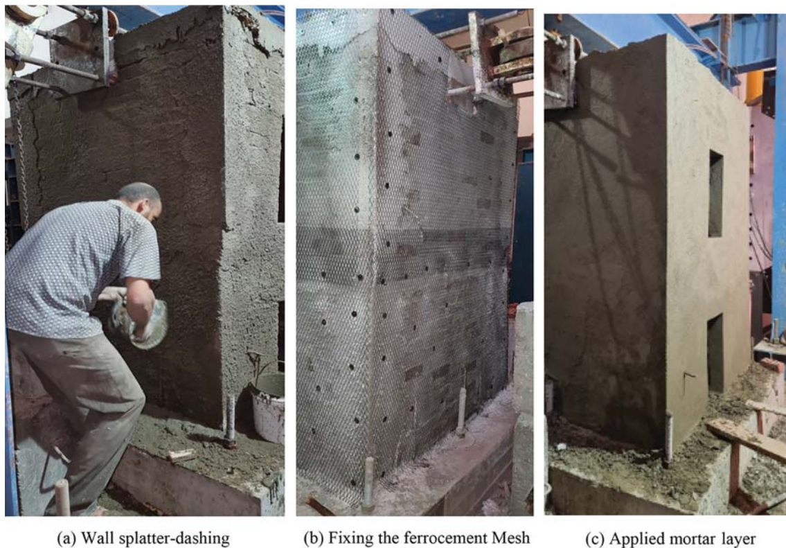
Fig. 4 Ferrocement’s retrofitting 3D assembly procedures
