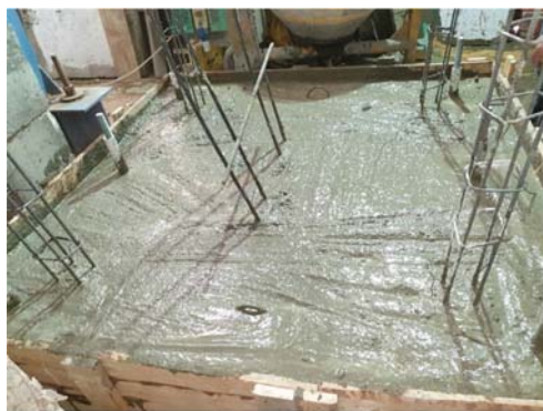
(a) Base footing and columns dowels
