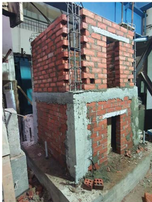
(c) Casting of R.C. columns/beams/slab of 1st level
