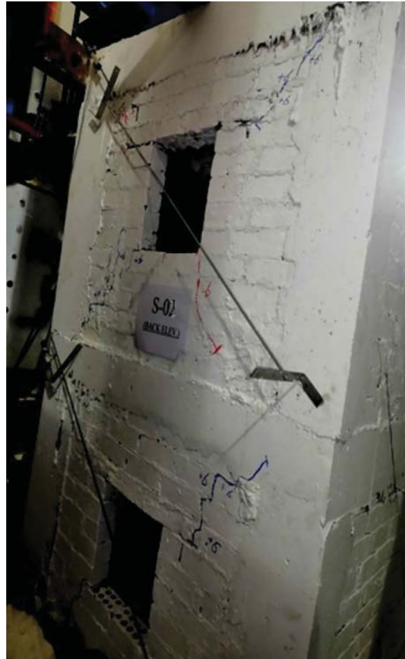
Fig. 10 The first obvious cracks S-01 (back)
