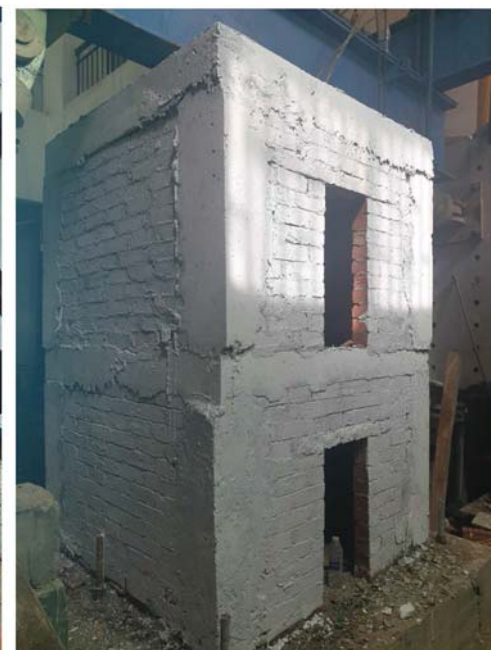
(d) the last instance of an un-strengthened assembly (S-01)
