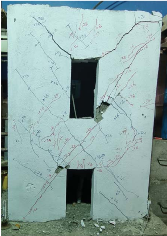
Fig. 17 Failure crack pattern S-02 (front)
